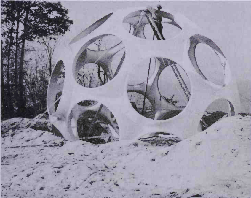
FIGURE 41. 26-foot-diameter Fly's Eye dome prototype
